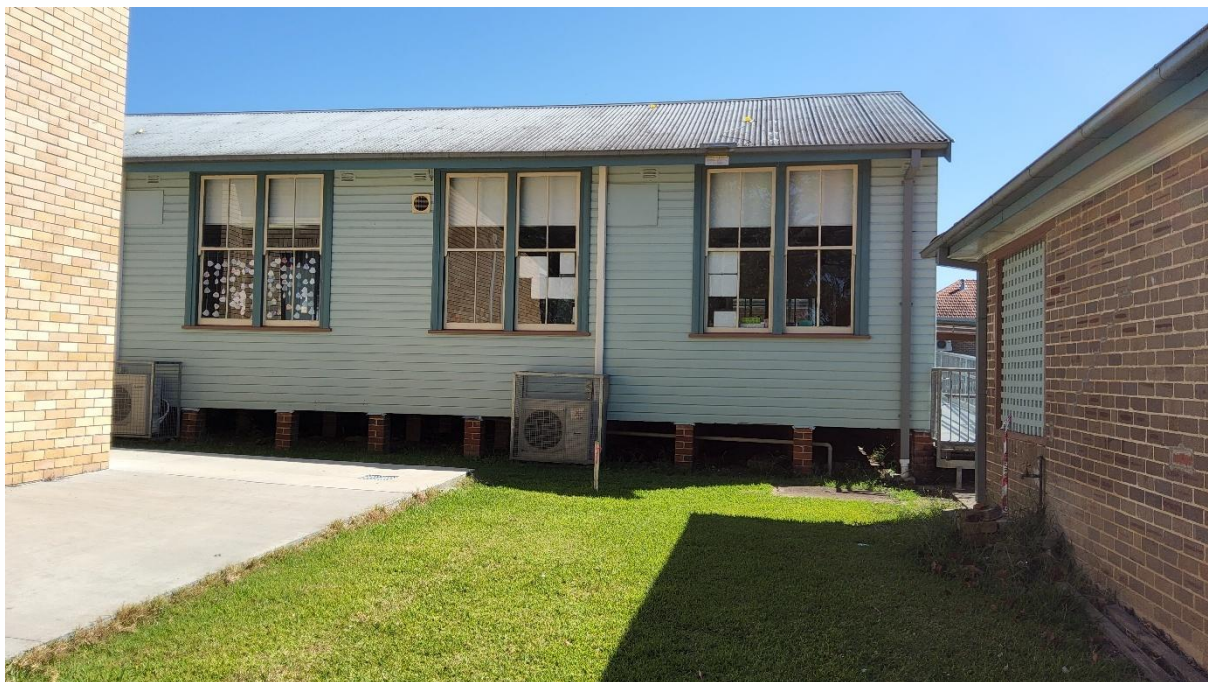
Plate 3. Older building on built on piers, newer building on left built on concrete slab. (Source: Heritage Now 2025)
